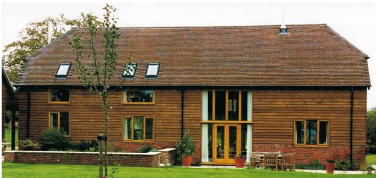
Figure 14 Rear view of the property
