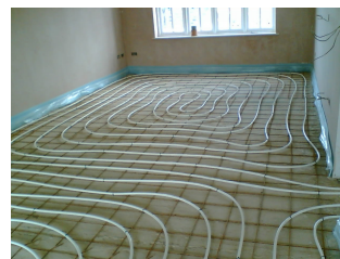
Structural Floor System
